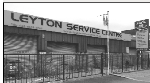
Leyton Service Centre - yet more flats
